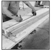
MEASURE AND MARK: Mark a guide line on top of 2"x 12" approximately 2-5/8" along each long edge.
