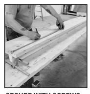
SECURE WITH SCREWS: Attach with deck or flathead wood screws at approx. 18" intervals along guide line.
