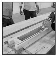
CLAMP & GLUE: Clamp both ends, then apply 3/16" to 1/4" bead of construction adhesive (PL400 or similar) to each support 2"x 4".
