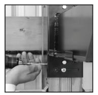
**SECURE SIDES: Right side first** — Fasten sides with screws though pre-drilled holes.
