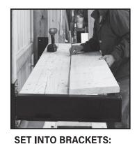
Set two shelving sections into each set of brackets, front and back.
